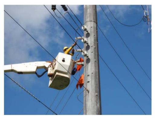
4) Structure 1 – KIUC crew cutting jumpers on structure 1 to de-energize the line.
