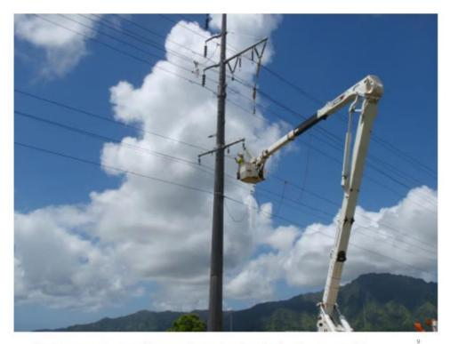
7) Structure 2 - Installing conductor in rollers (other than neutral.)
