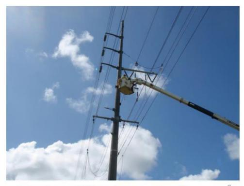
9) Structure 2 – Installed lower transmission arm and assemblies.
