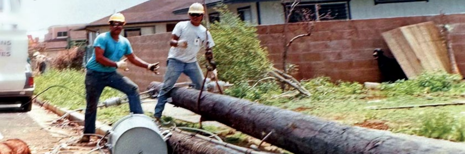
Kaua'i Electric line crews make repairs following Hurricane 'Iniki in 1992.
