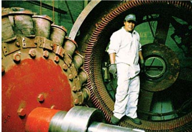
Figure 8-11. Waimea Mauka Powerhouse Generator Maintenance (Source: Hawaii Business Magazine, Nov. 2003).
