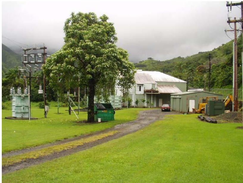
Figure 8-5. Existing Wainiha Hydropower Plant.
