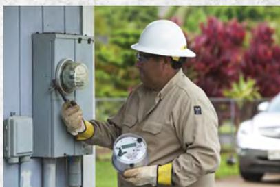
Installation of advanced metering infrastructure (AMI) is completed.
