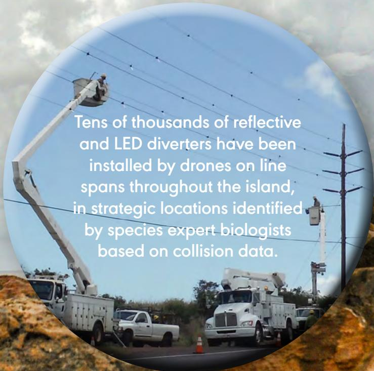
Tens of thousands of reflective and LED diverters have been installed by drones on line spans throughout the island, in strategic locations identified by species expert biologists based on collision data.
