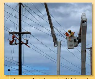
Line reconductoring work in Kekaha and Mānā is completed to support the new PMRF substation construction
