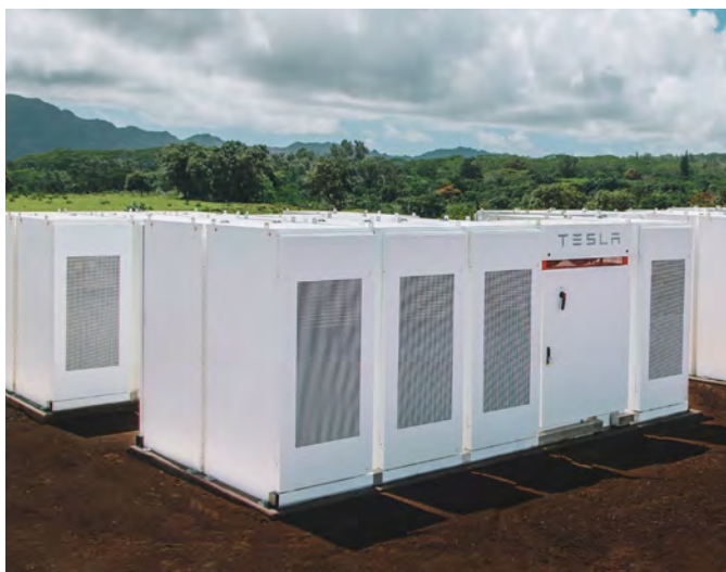
The 52 MWh Tesla Powerpack system will help power Kaua'i in the evening when loads are greater.
