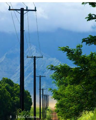
It is important to know that the higher on the pole you go, the more dangerous the wires become. The exposed power lines at the top carry the highest voltage.
