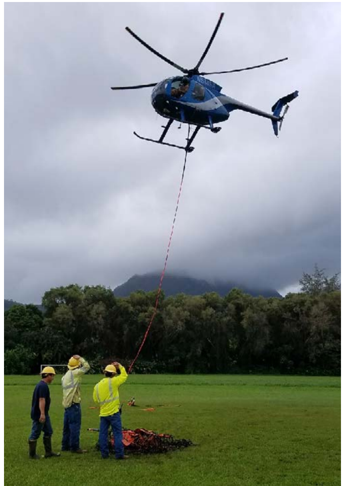
KIUC line crews await helicopter transport to Wainiha.
