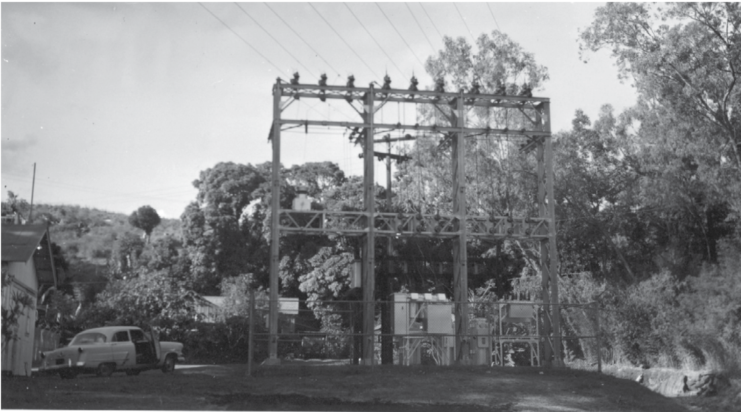
New switchyard at Kalaheo hydro plant, 1956.
