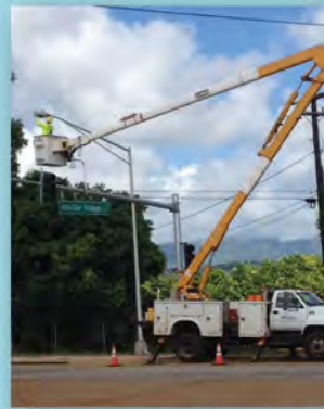
January 2017: Kaua'i is the first county in the state to convert all of its streetlights to LED technology, offering reduced energy use, a longer lifespan and lower maintenance costs.
