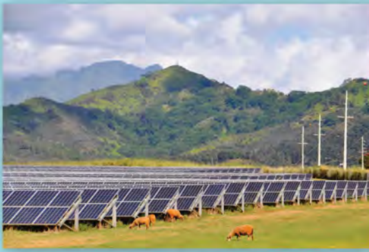
August 2014: KIUC's Kōloa Solar project comes on line, serving nearly 6% of Kaua'i's energy needs and reducing fossil fuel consumption by 1.7 million gallons a year.
