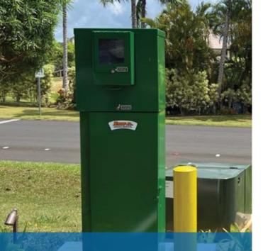
The installation of a new transformer near the old transformer was required to meet the increased electricity load.
